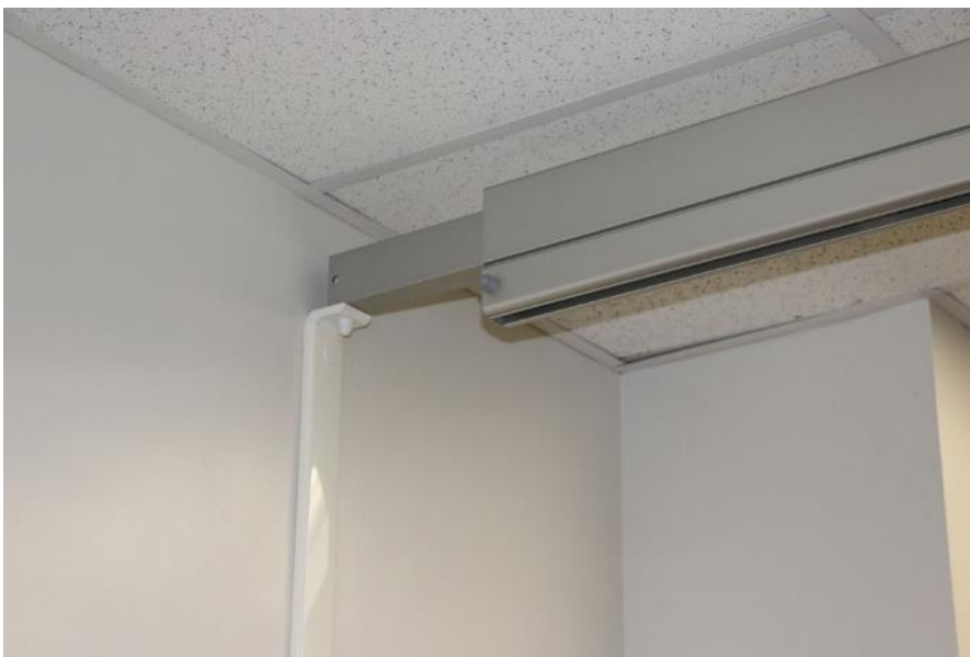
Figure 2-2 – wall-mounted end support of track
