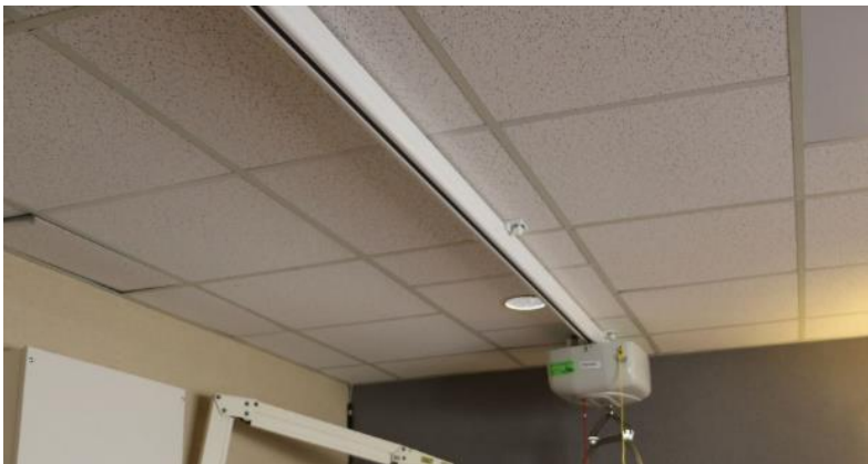
Figure 2-1 – straight track with above-ceiling support
