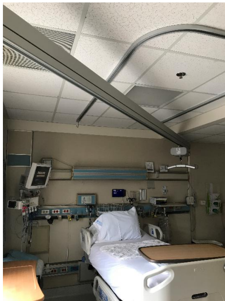
Figure 34 – straight track at angle over bed
