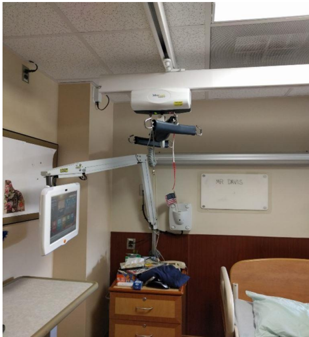
Figure 5 – monitor on retractable boom arm
