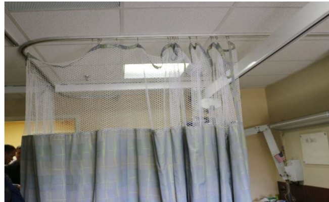
Figure 8 – privacy curtain showing rail and lift interaction
