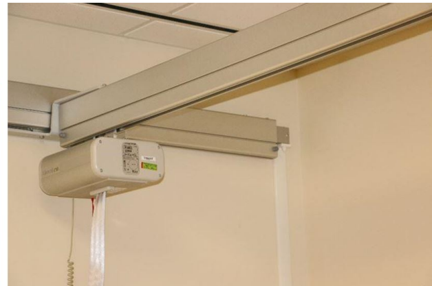
Figure 37 – wall mounted fixed rail parallel to wall
