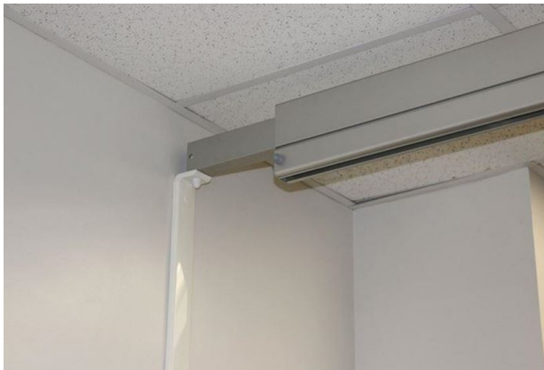
Figure 36 – wall mounted fixed rail perpendicular to wall
