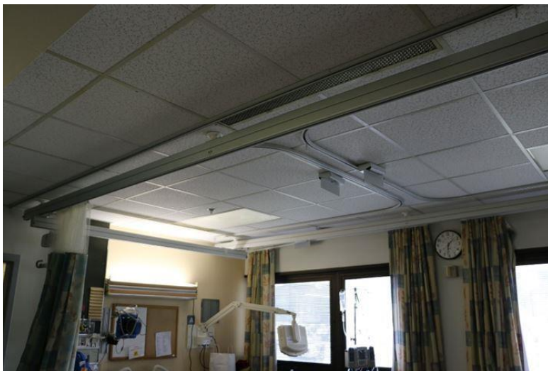
Figure 27 – privacy curtains inside lift access area
