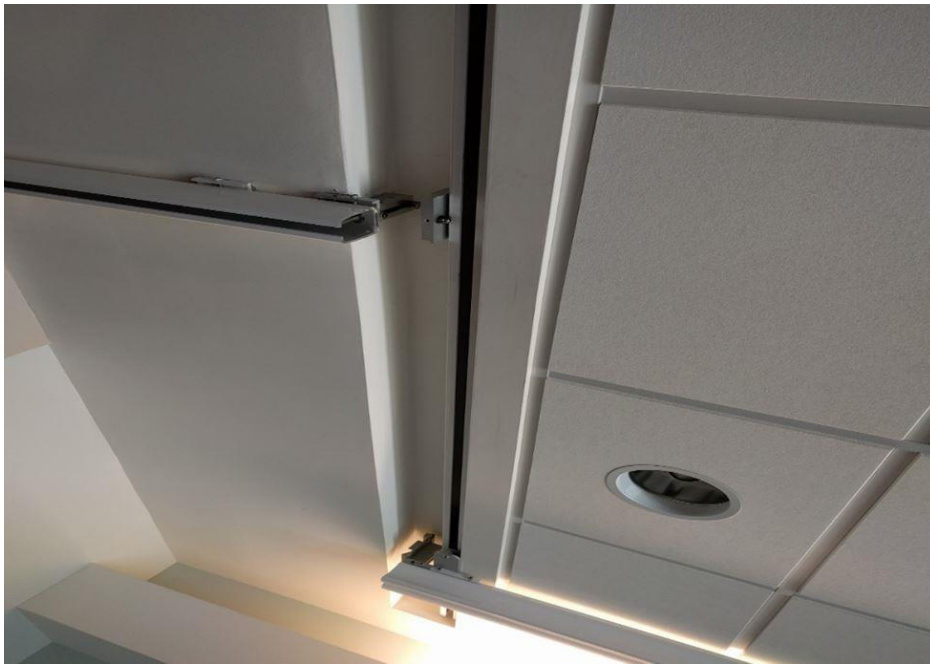
Figure 4 – recessed track with junction for connection to single-rail into bathroom
