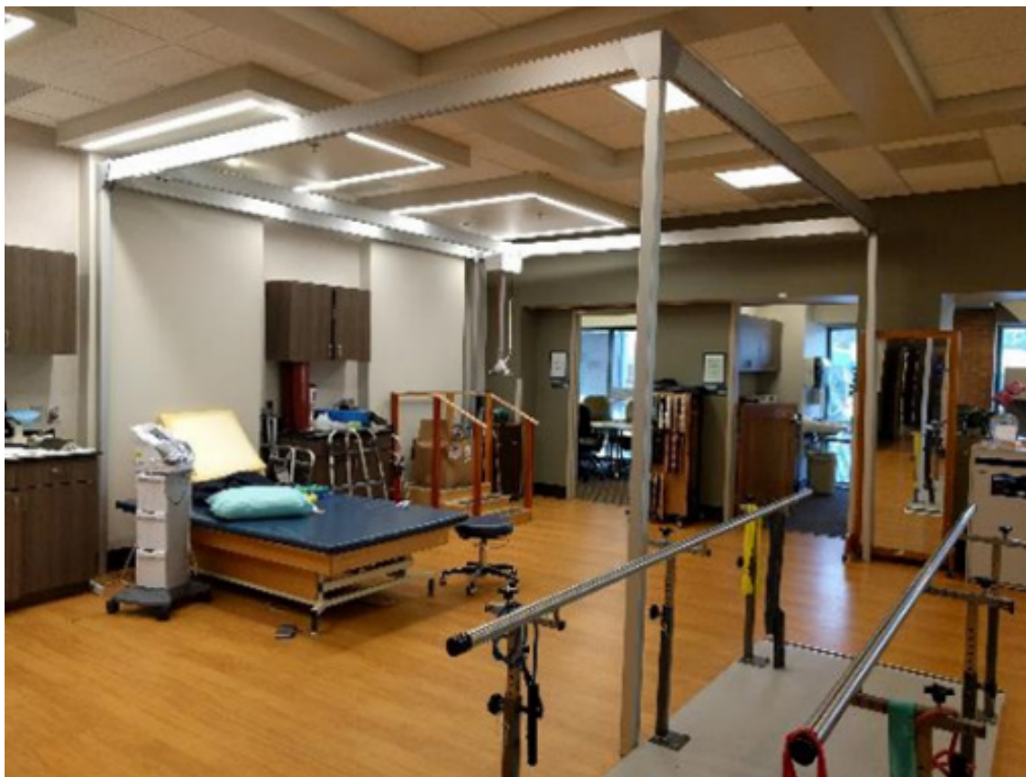
Figure 2-8 – 4-point gantry lift over PT exam table
