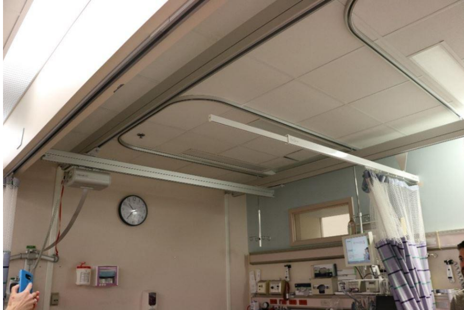
Figure 22 – PACU with telescoping privacy curtain
