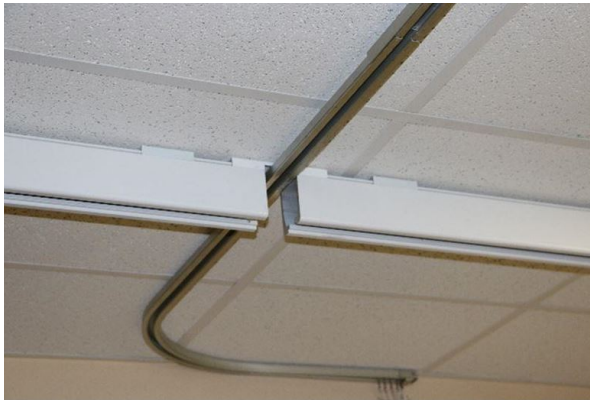
Figure 7 – gap in fixed rail for movement of privacy curtain
