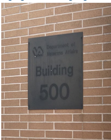
Figure 1-3 (Above) Over time, a buildup of dirt and oxidization can obscure a sign's message, making it difficult to read.
