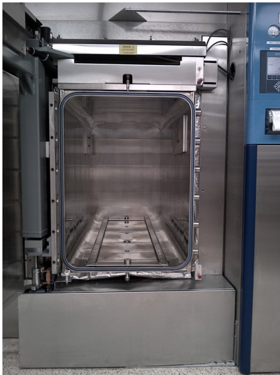
Figure 13: Front Loading Steam Sterilizer (SPS)
