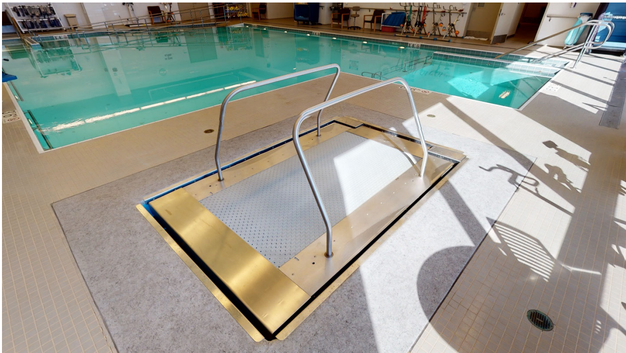
Figure 3.6 The Treadmill Pool at the New Orleans VAMC includes jets for resistance and cameras to observe underwater motion.
