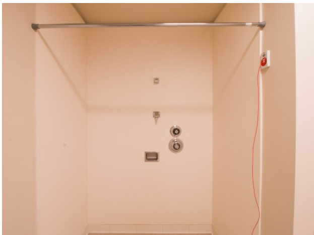
Photos of Behavioral Health rooms with anti-ligature fixtures and accessories.
