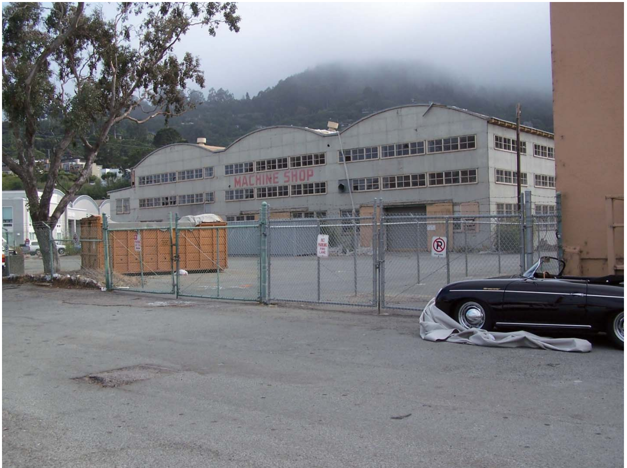
Name: Marinship Machine Shop Address: 25 Liberty Ship Way, Sausalito, Marin County CA Photographer: Bonnie Bamberg Date: July 2009 View: Main (front) Façade Camera Facing West Photograph # 2.9. 1
