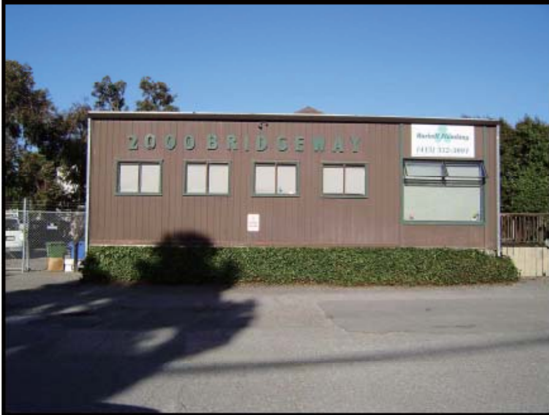
Picture # 8 2000 Bridgeway, Sausalito CA Burkell Plumbing modular building. Constructed 2000, Age: 10 years View: Front (East) Façade of the building Photographer facing North
