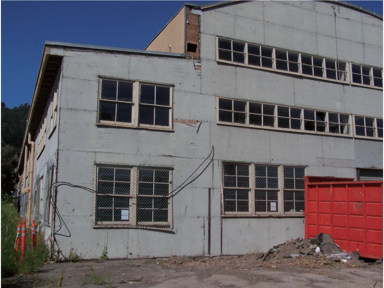
Name: Marinship Machine Shop Address: 25 Liberty Ship Way, Sausalito, Marin County CA Photographer: Bonnie Bamburg Date: July 2009 View: Front (East) Façade- Office addition, 1943 Camera Facing Southwest Photograph # 2.9. 2
