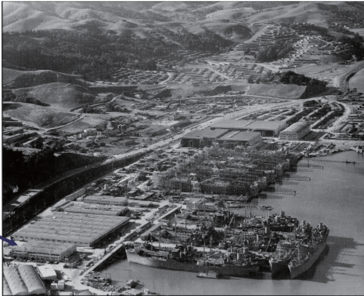
Photograph # 5 Marinship facility c. 1943, Arrow locates the Machine Shop Building Source: Marinship Archives, Bay Model Building, Sausalito
