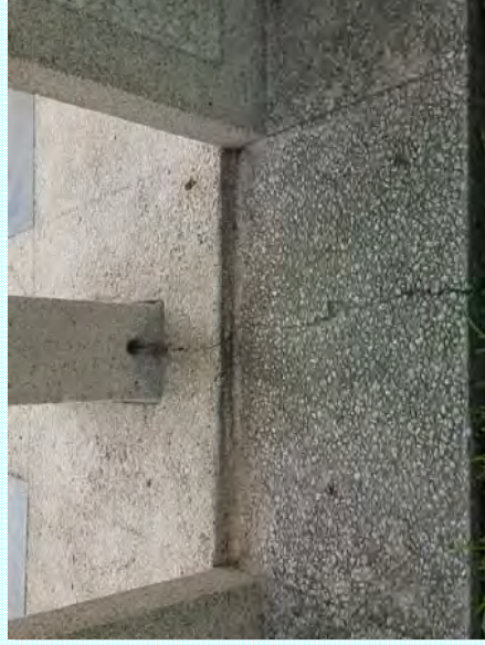
Photo: G—Flatwork cracking and spalling at the outside columns
