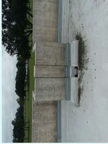
Photo: C—Biological staining on the inside of the upper panels
