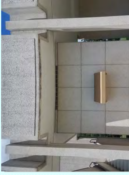
Photo: H—Staining at the bottom of the upper panels
