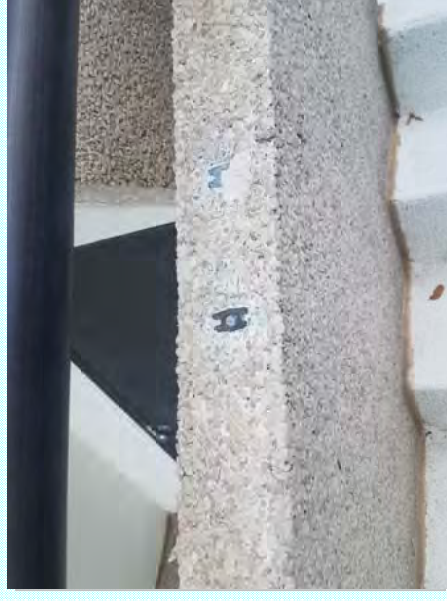
Photo: D—Exposed steel fasteners at the top of upper panels
