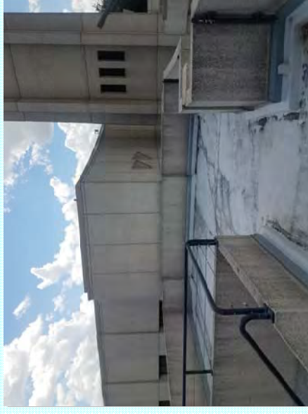
Photo: B—Biological settlement on upper deck along the perimeter
