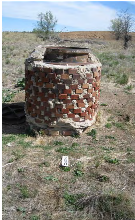
Figure 7. HRA-FL1, raised brick and mortar manhole cover.
