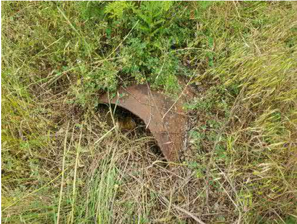
Photo 7 Metal Drainage pipe embedded in ground.
