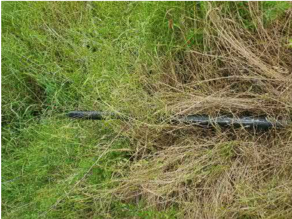
Photo 8 PVC Drainage pipe embedded in the ground.
