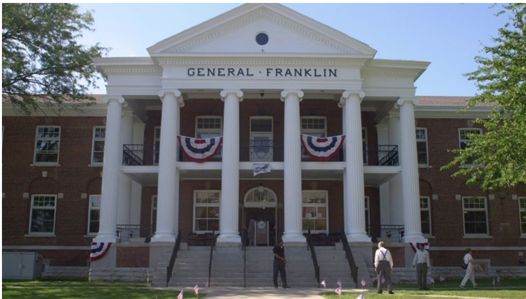
Figure 11: Building 412 at Dayton after project completion, 2021.
