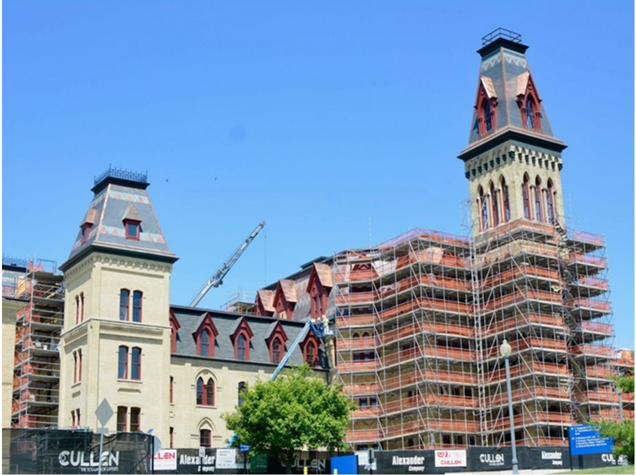
Figure 9: Milwaukee VAMC’s Old Main during rehabilitation.
