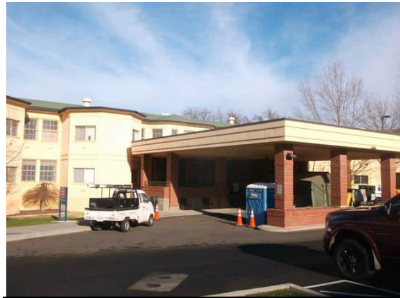
Photo #4: Looking northeast at Building 74
