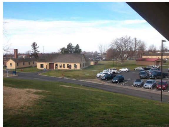
Photo #32: Looking northeast at the north adjoining Buildings 63 and 65 and Parking Lot #1
