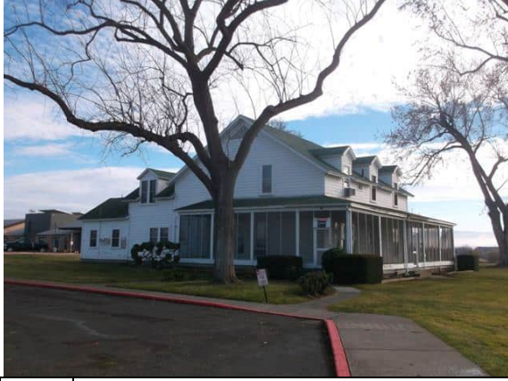
Photo #1: Looking southeast at Building 1
