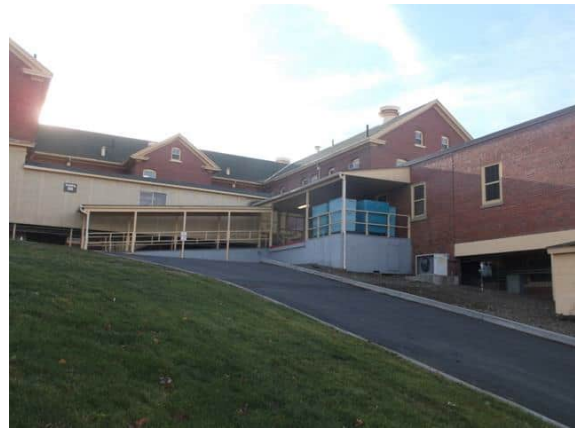
Photo #12: Looking south at Buildings 80 (right) and 69 (left and center)
