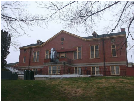
Photo #11: Looking southwest at Building 78
