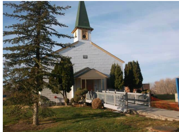
Photo #40: Looking northwest at the campus chapel (Building T-7)
