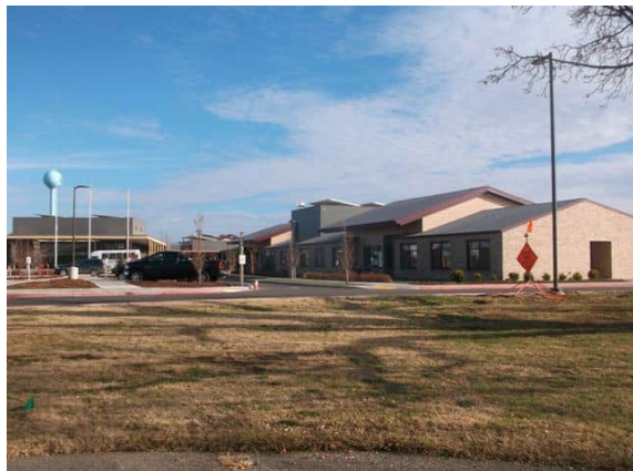
Photo #35: Looking east at the east adjoining State Veterans Home
