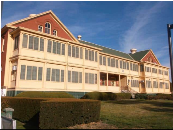
Photo #3: Looking northeast at Building 69
