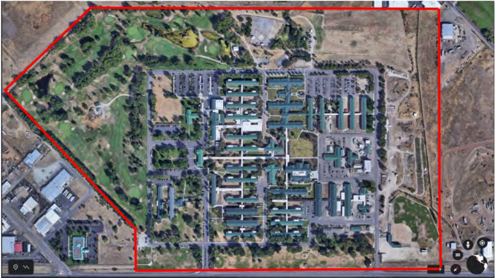
Figure 1-2 Southern Oregon Rehabilitation Center & Clinics, White City, Oregon
