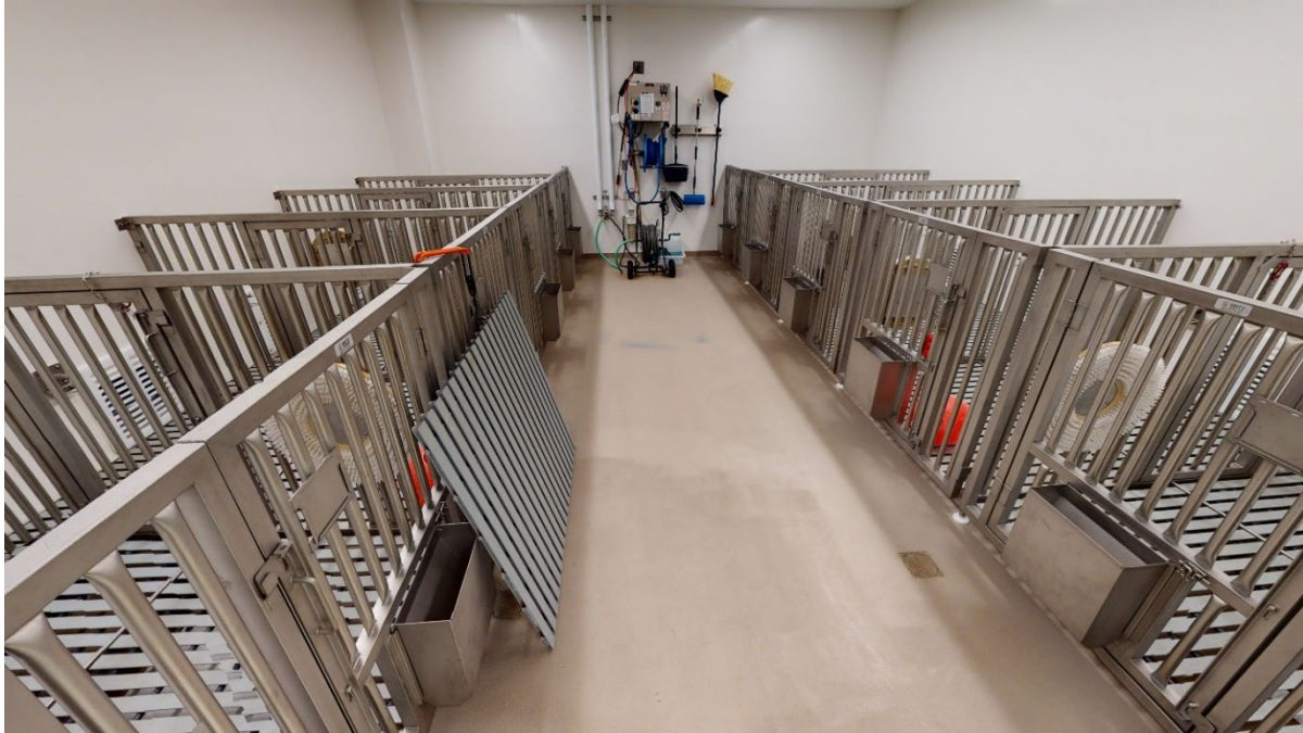
Image A.7 Cages in the Large Animal Holding Room at the Rocky Mountain VAMC R&D Facility include openings for social interactions and open grate flooring for cleaning.
