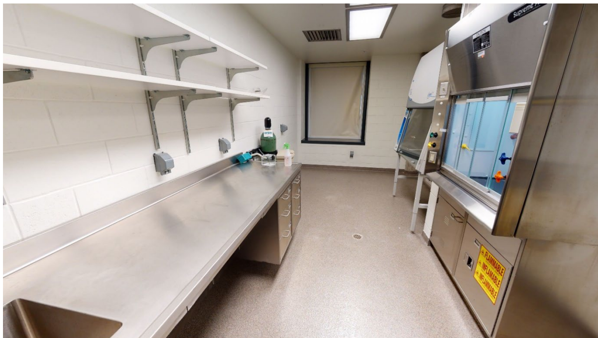
Image A.21 A VMU General Procedure / Treatment Room at the New Orleans VAMC R&D Facility contains stainless steel cabinetry, a biological safety cabinet, and a fume hood.
