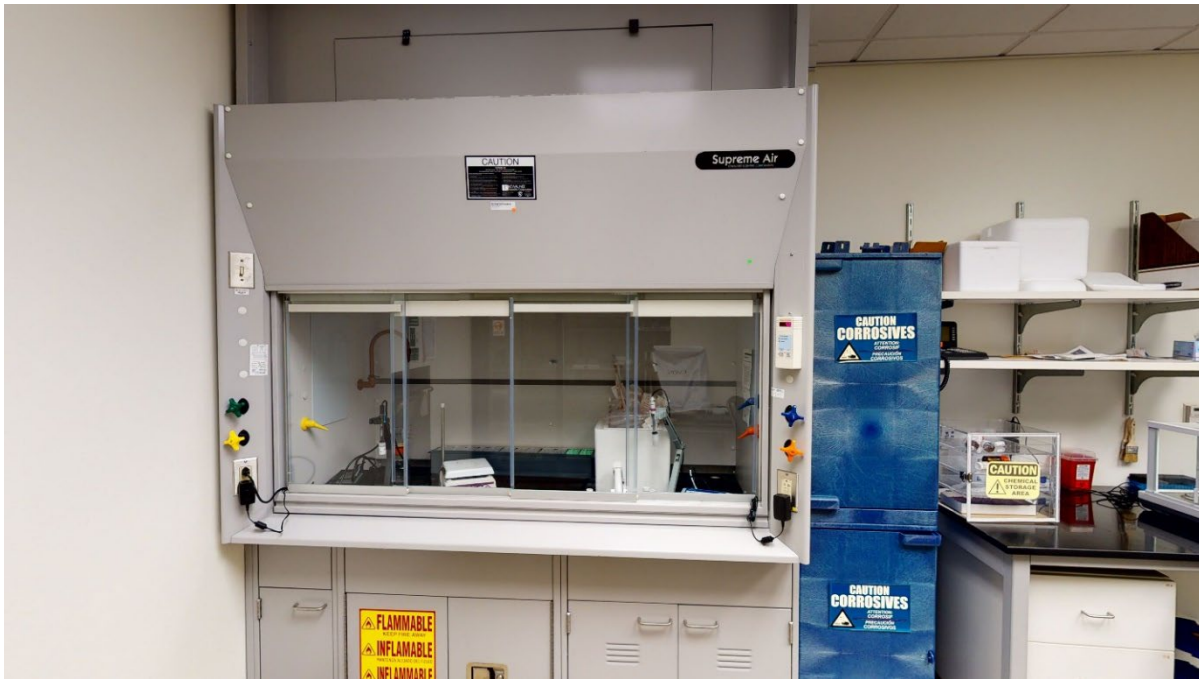
Image A.16 A fume hood at the New Orleans VAMC R&D Facility is located next to a corrosive storage cabinet, and share ventilation.
